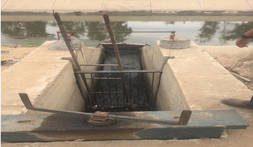
Figure 6.3: Water Intake from Al-Kassara Tertiary Canal directly to Al Dahra farm in Al Salheya
